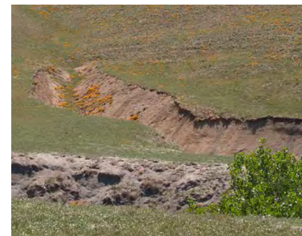
[Figure VII.47 GULLYING AT BRONCO CANYON, TEJON RANCH.]
