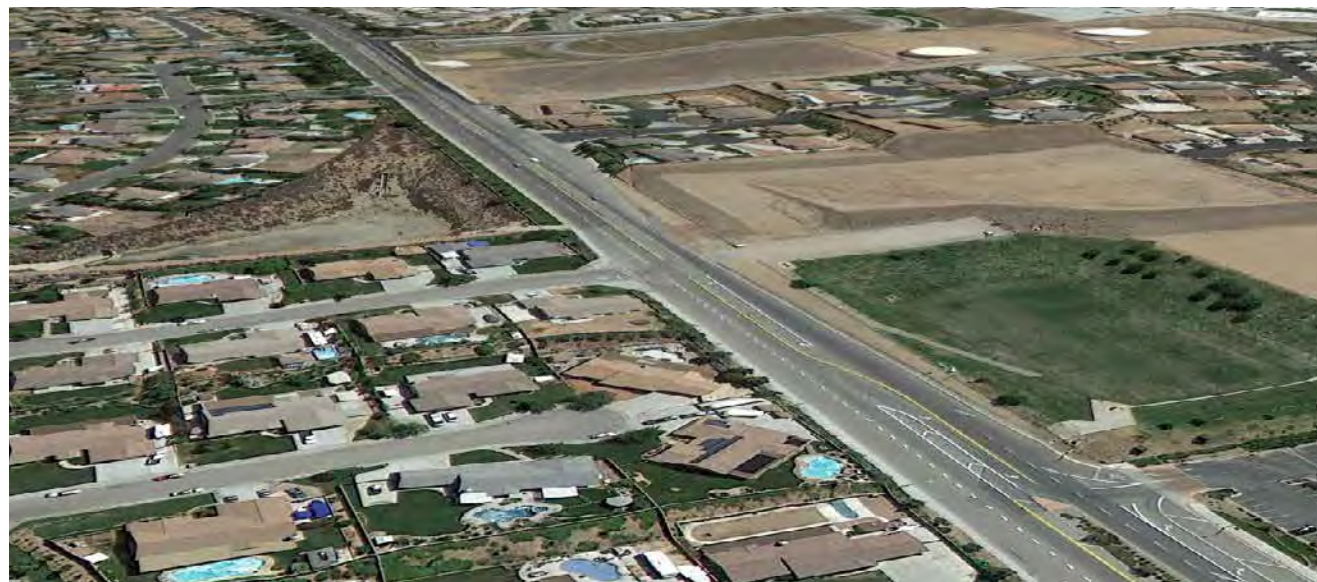
[Figure VII.50] TWO DETENTION BASINS IN PALMDALE, INCLUDING QUINONES PARK. Source: Google]
